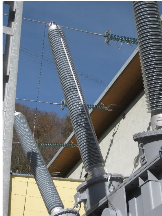
Figure 6: Example of shortest-braid connection concept - measurement cables (black) are connected to the bushing terminal and the grounding braid to the terminal and bushing flange
