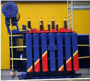
Figure 2: 6,5 MVA, 47 kV/27,2 kV power transformer
