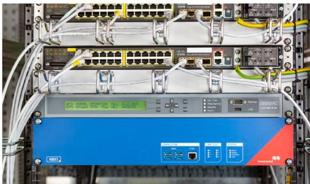
Figure 4: StationGuard installed in a greenfield 110kV substation, 2019
