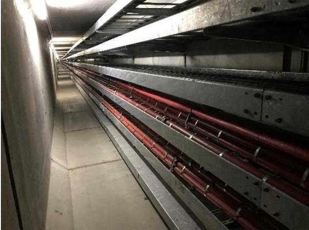
Figure 8 - 500 m, 6-kV-Cable system with 2300 A rated current
