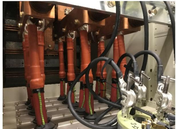
Figure 2 - Parallel connection of single-core medium-voltage cables to a switchgear system
