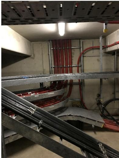
Figure 5 - Various medium-voltage cable routes in the cable basement
