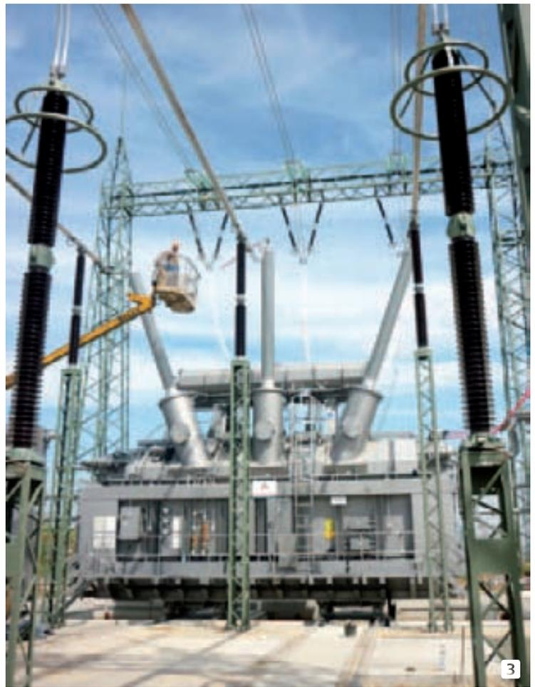
**1** Primary testing device for generating up to 2,000 A with connection cables to provide a primary supply. **2** Current transformer testing with the CT Analyzer on a current transformer in the bushing of a 30 kV E-reactor. **3** Current transformer testing with the CT Analyzer on a current transformer in the high-voltage bushing of a 380 kV power transformer.
