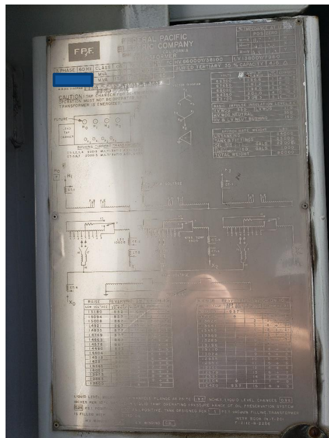
Figure 8: Nameplate Example Showing Presence of Tie-In Resistor
