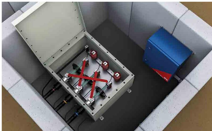
The cement boxes protect the HFCT sensors and data acquisition unit against ground water and dust.
