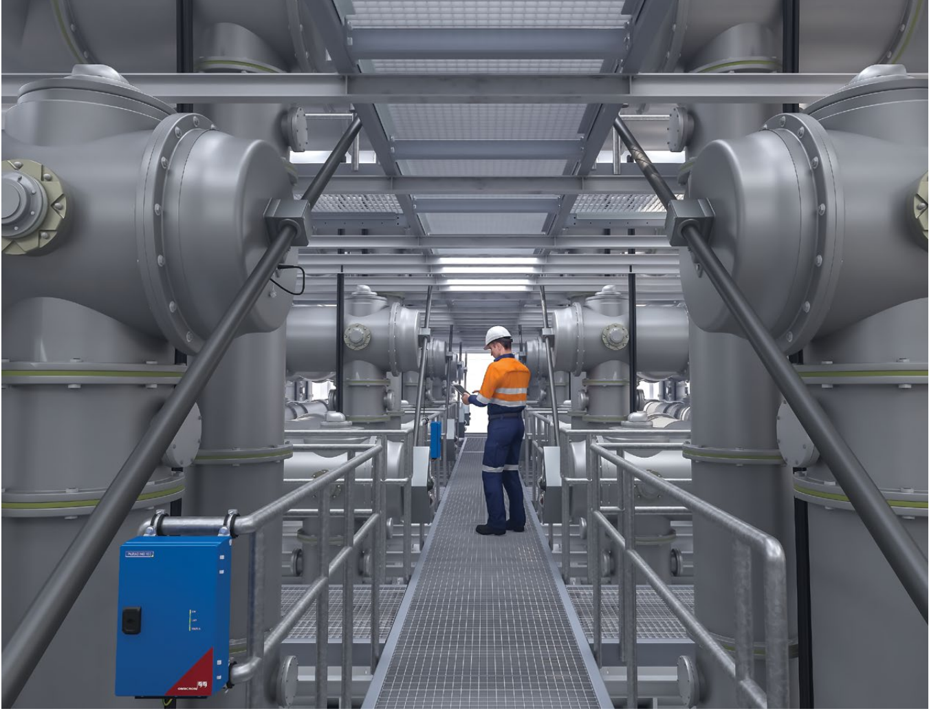
PARADIMO 100 devices communicate via standard network protocols. Multiple monitoring points facilitate trending, defect detection, and classification for reliable risk assessment in GIS and GIL.
