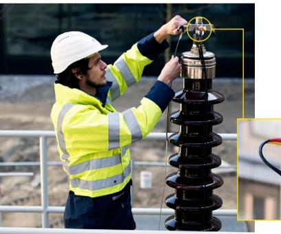
Due to the special design of the bushing clamps a reliable contact is achieved.
