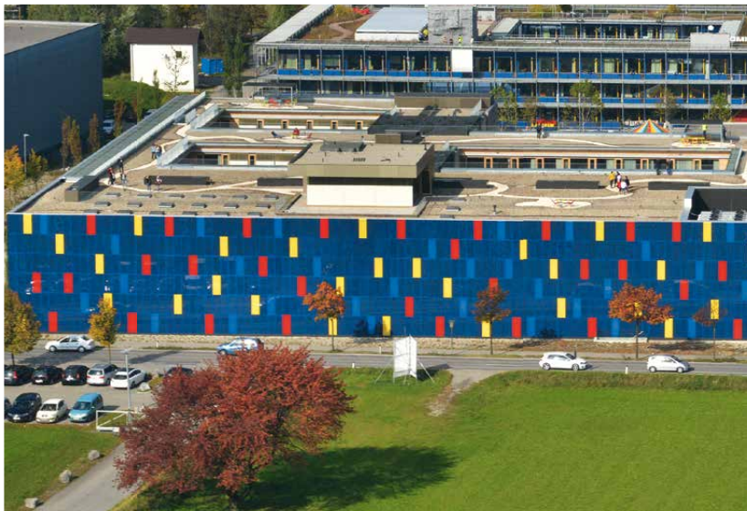
780 m 2 / 8,396 ft 2 of photovoltaic panels are installed at the frontside of OMICRON's office in Klaus.
