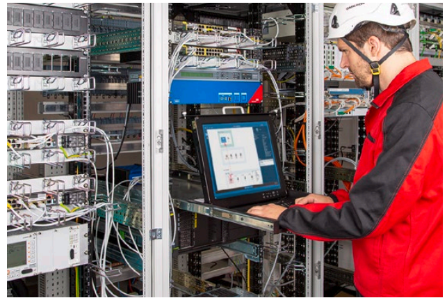
Figure 3: StationGuard imports the SCL (System Configuration Language) file of the substation to create a complete system model
