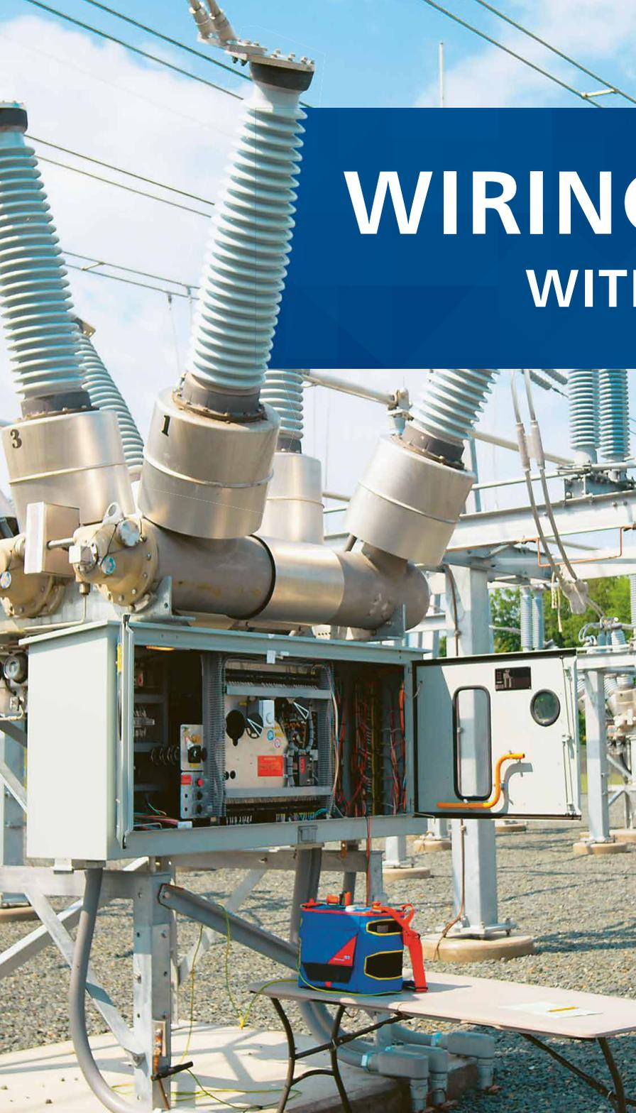
Having the correct polarity for voltage and current transformer circuits is essential if the protection relay that is connected to them is going to function properly.
