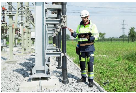
Quick and easy Step and Touch Voltage measurement using HGT1 and PTM software
