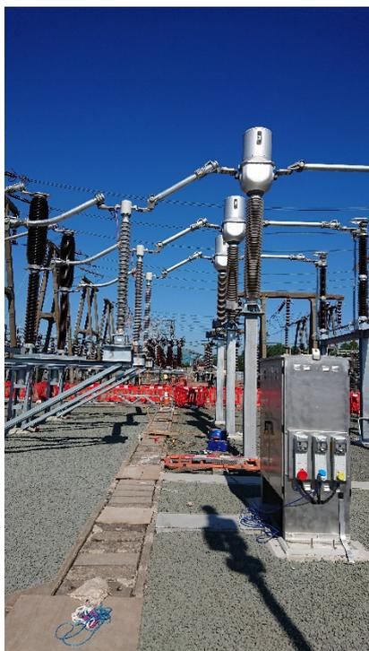
**Fig. 7:** Test with the CPC 100 in which the test current is driven by a conventional and a non-conventional transformer
