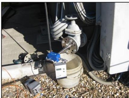
Figure 4: Drain valve sensor for insertion temporary into the transformer
