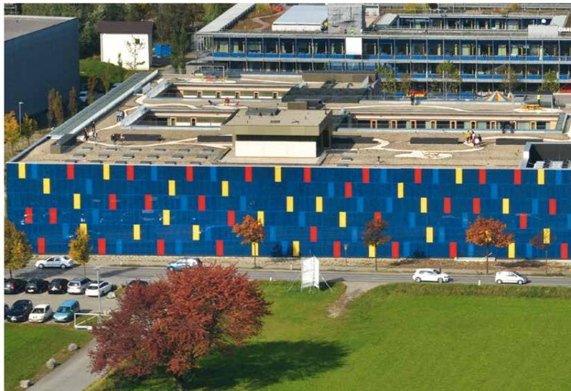
780 m<sup>2</sup> / 8,396 ft<sup>2</sup> of photovoltaic panels are installed at the frontside of OMICRON's office in Klaus.
