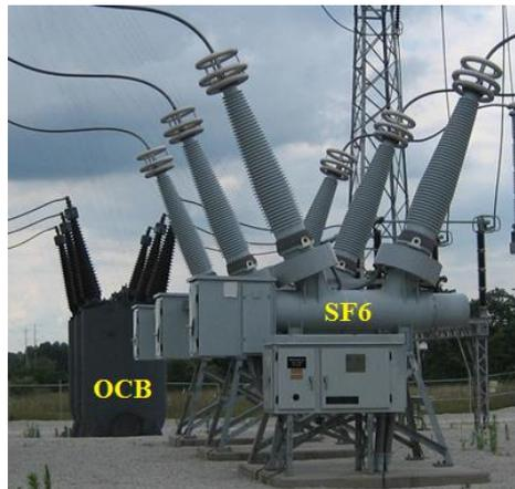
Figure 1 - Bulk OCB vs. Dead Tank SF6
