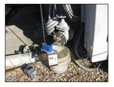
Figure 4: Drain valve sensor for insertion temporary into the transformer
