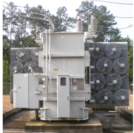
Bushings are a necessary component of a power transformer, but they are one of the transformer's main weaknesses.
