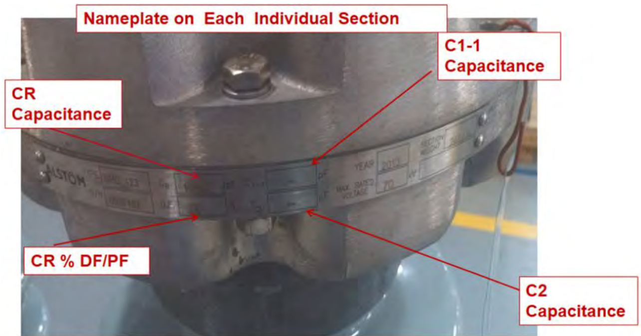
Figure 25: Capacitor Stack Nameplate of Alstom Type OTCF 300 CCVT
