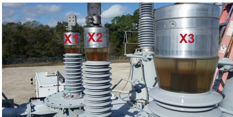
Figure 11 – Sight Glass Comparison for the Three ABB O+C 72kV Bushings
