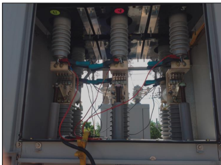
Figure 16 – Leads connected directly across the vacuum bottles
