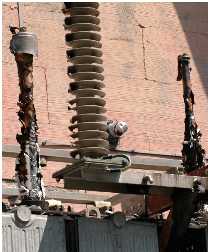
Exploded bushings due to aging insulation on a power transformer
