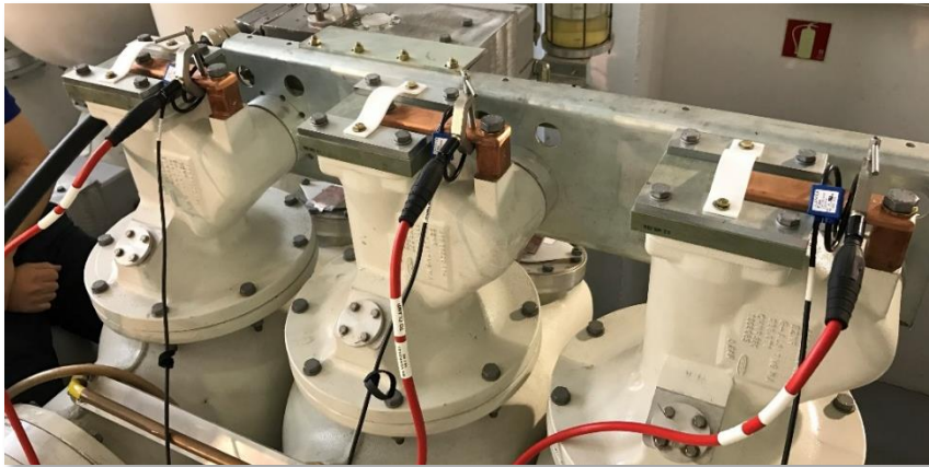
Figure 17 - GIS 245 kV with three enclosures, one for each phase.
