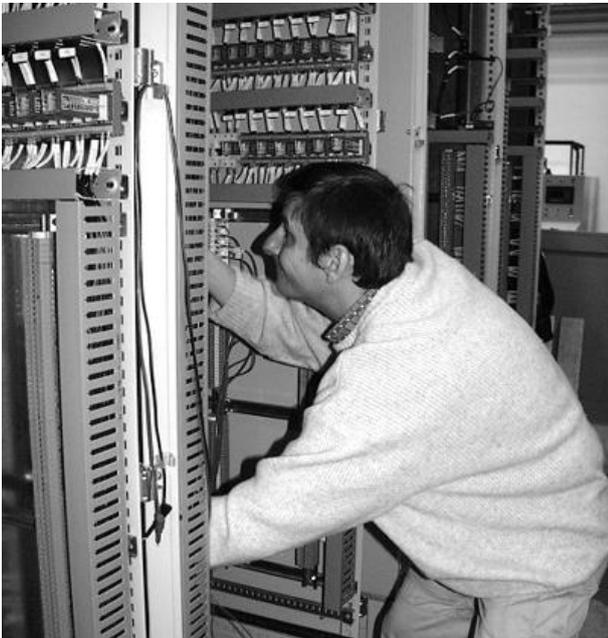
Figure 14: Time-consuming point-to-point testing in the copper-wiring era, before fiber glass
