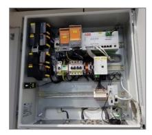
Figure 5 Remote signaling and control using ABB FIONA
