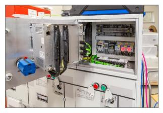
Figure 8 ABB sensor test adapters in the low-voltage compartment
