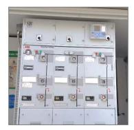
Figure 6 ABB SafeRing AirPlus 20 kV switchgear
