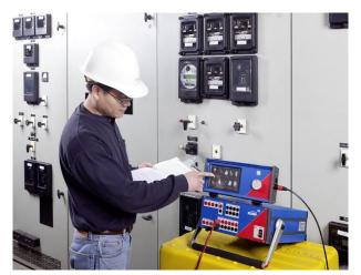
Figure 15: Quick manual testing with CMControl for simple test tasks
