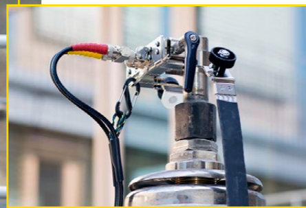
Due to the special design of the bushing clamps a reliable contact is achieved.
