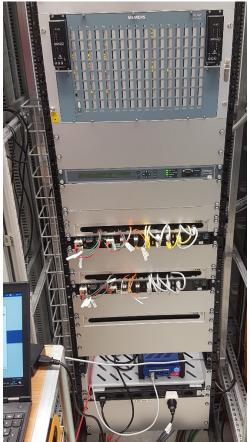
Figure 3 Installation in 110kV substation of CKW using the mobile platform variant of StationGuard
