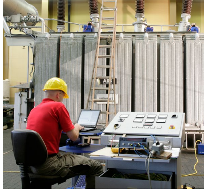
Off-line PD measurements being performed with the MPD 600 on a transformer during factory acceptance testing.
