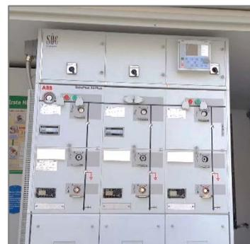
Figure 6 ABB SafeRing AirPlus 20 kV switchgear
