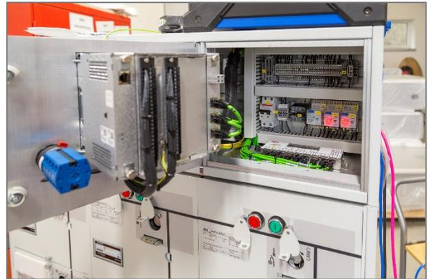
Figure 8 ABB sensor test adapters in the low-voltage compartment
