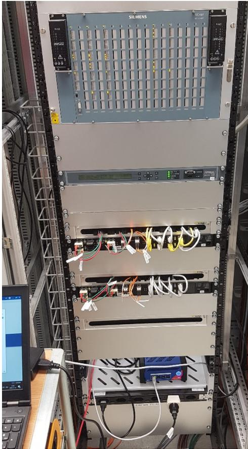
*Figure 3 Installation in 110kV substation of CKW using the mobile platform variant of StationGuard*
