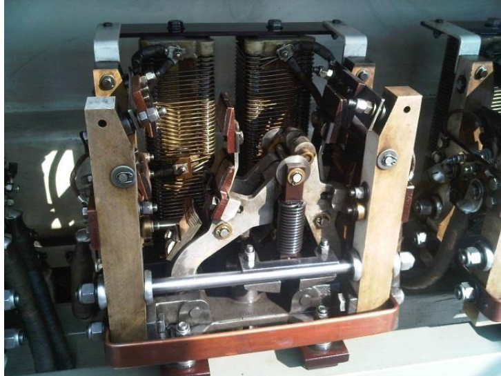
Figure 12 – Diverter Switch
